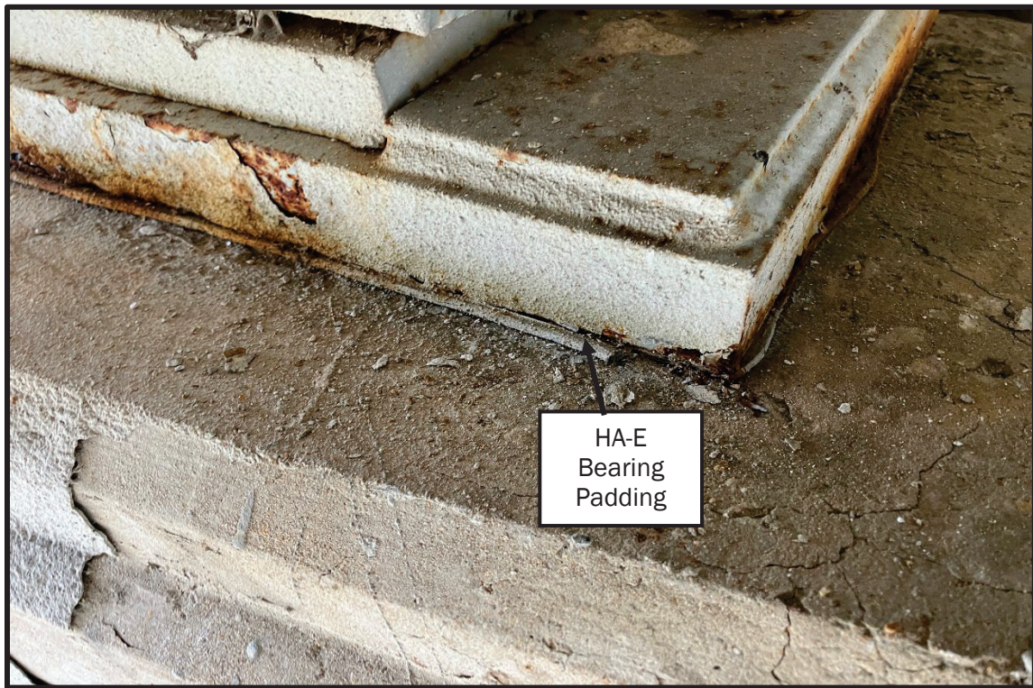
Photo 5: View of HA-E from under the north end of the bridge.
