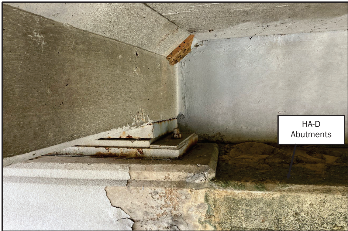
Photo 4: View of HA-D under the north end of the bridge.
