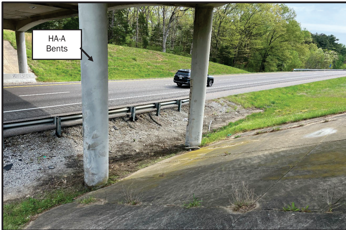
Photo 2: View of HA-A from the southern portion of the bridge.
